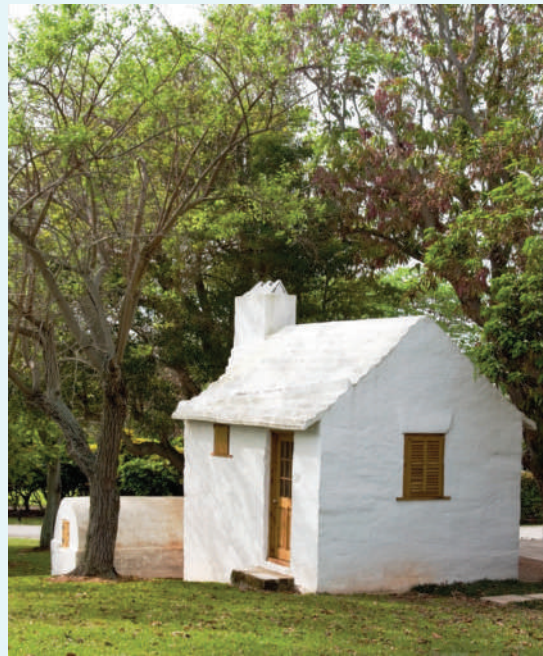
Tiny old Bermuda cottage with limestone roof - to catch water in the separate raised water tank below the house.
