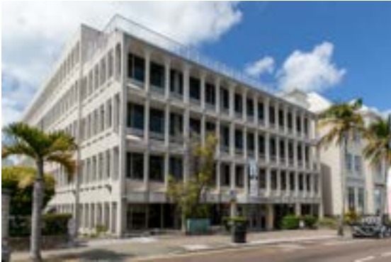
The usable space within this building is set back from the primary façade to reduce direct exposure to the sun and the need for mechanical cooling.
