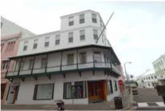
An example of a building responding to its location on a corner lot through using an additional storey to define the corner, a wrap-around veranda and a splayed corner.
