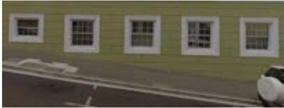
The design of this building has not recognised the topographical changes of the site and has instead reduced the size of a window to maintain a linear approach..
