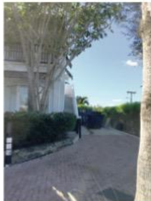
Service and Maintenance Area
